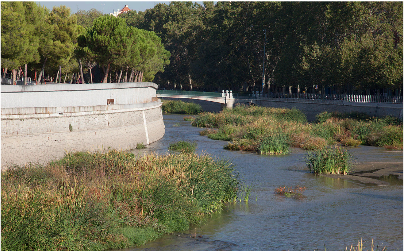
Figure 3 – Evolution of the urban reach of the Manzanares River near the historical Toledo Bridge: (a) by the early 20th century, showing the characteristic patterns of the near-natural multi-thread river channel; (b) in the 80s, after the canalization of the river and the construction of motorways along its banks; (c) in the early 21th century, after the motorways burial and the construction of a huge river park, but still with the weirs closed along the rivercourse; (d) after the full opening of the weirs and the allowance of a seminatural dynamics inside the limited space of the river (Photo sources: Madrid City Council and CEDEX).
