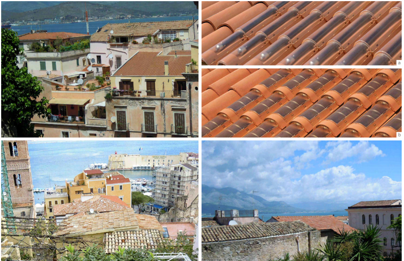
Figure 4 – Example of pitched roofs: a) Thermal solar system integrated into tiles; b) Photovoltaic system integrated into tiles.
