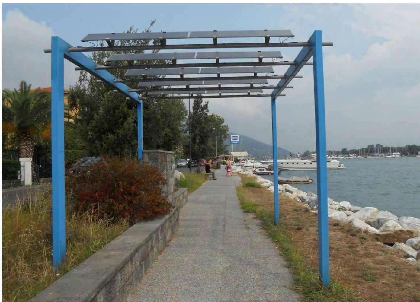
Figure 2 - Ameglia (La Spezia, Italy). One of three prototypes of stand-alone photovoltaic shelter made in 2004, as part of the Italian German PVACCEPT research project funded by the European Commission. This project is based on the integration in the architectural historic environment and landscape (photo R. Valente).
