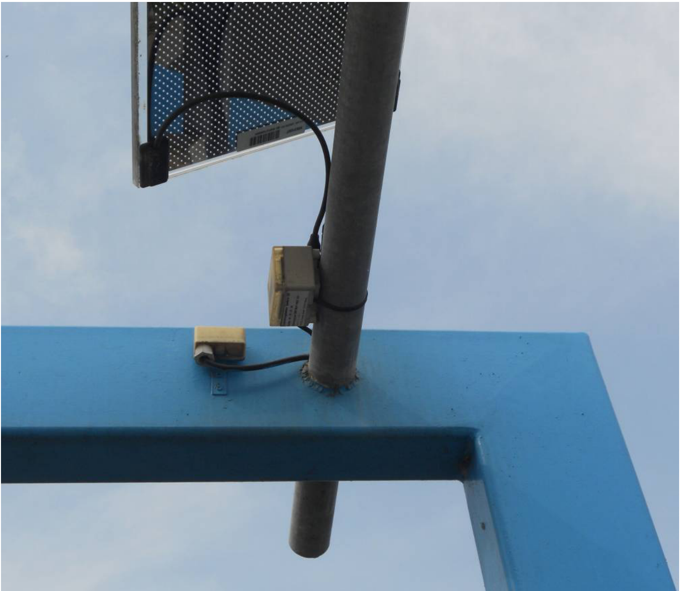
Figure 3 – Ameglia (La Spezia, Italy). Detail of photovoltaic trellis wiring. Five 2.40 m x 0.30 m module strips for each pergola facing south / east at an angle of 30 ° above the horizon, support the semi-transparent thin film with a pattern of 10% of holes which produce up to 240 Wp (photo R. Valente).
