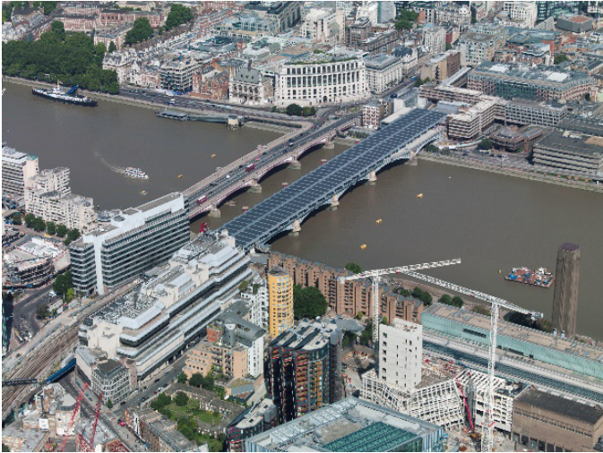
Solar Century, Blackfriars Bridge solar roof, London UK, 2014.
