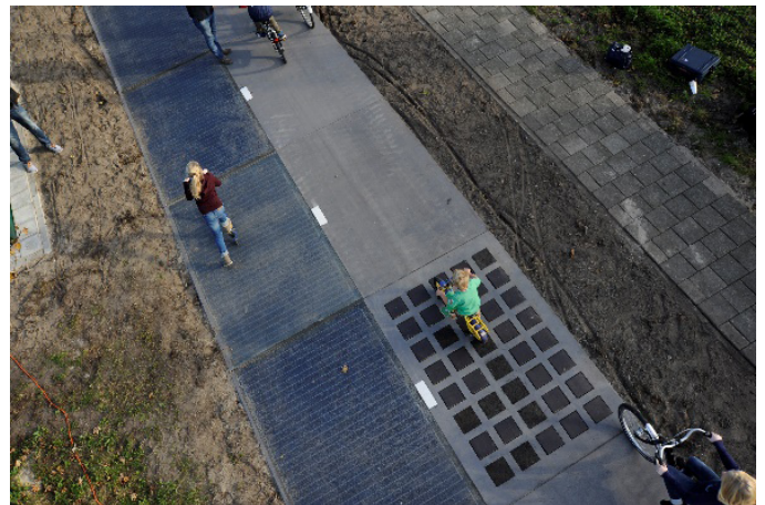
TNO, SolaRoad, Prefabricated PV system for urban paving, Amsterdam NL, 2014.
