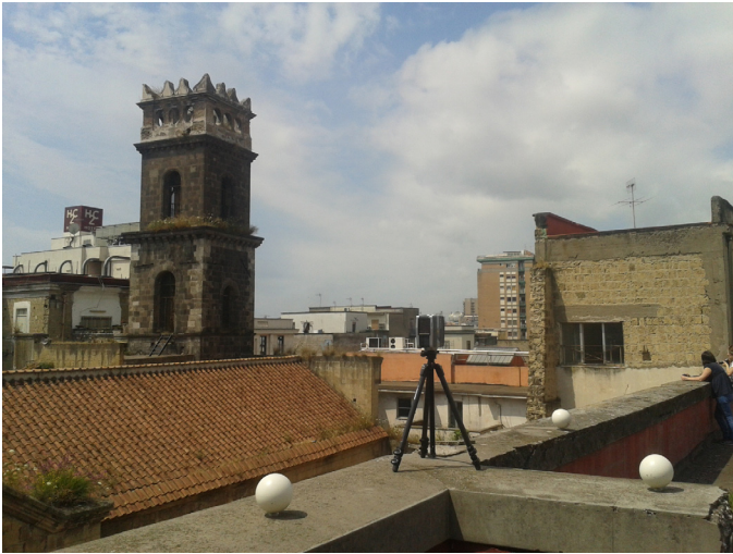
Figure 2 – Data acquisition of external facades with laser scanner using spherical target.
