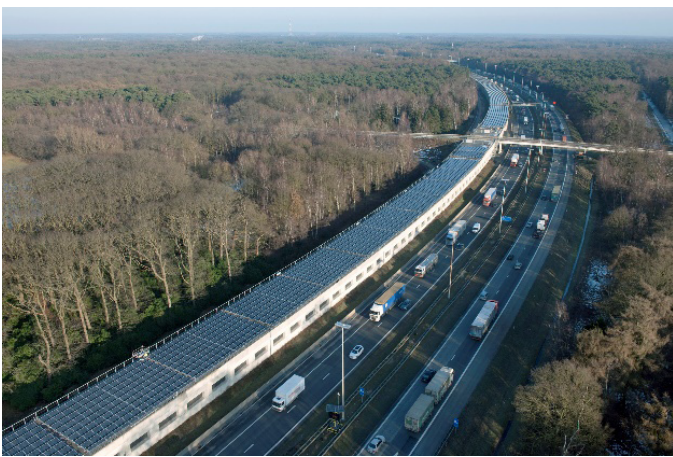
Infrabel and Enfinity, Solar tunnel, Brasschaat BE, 2011.
