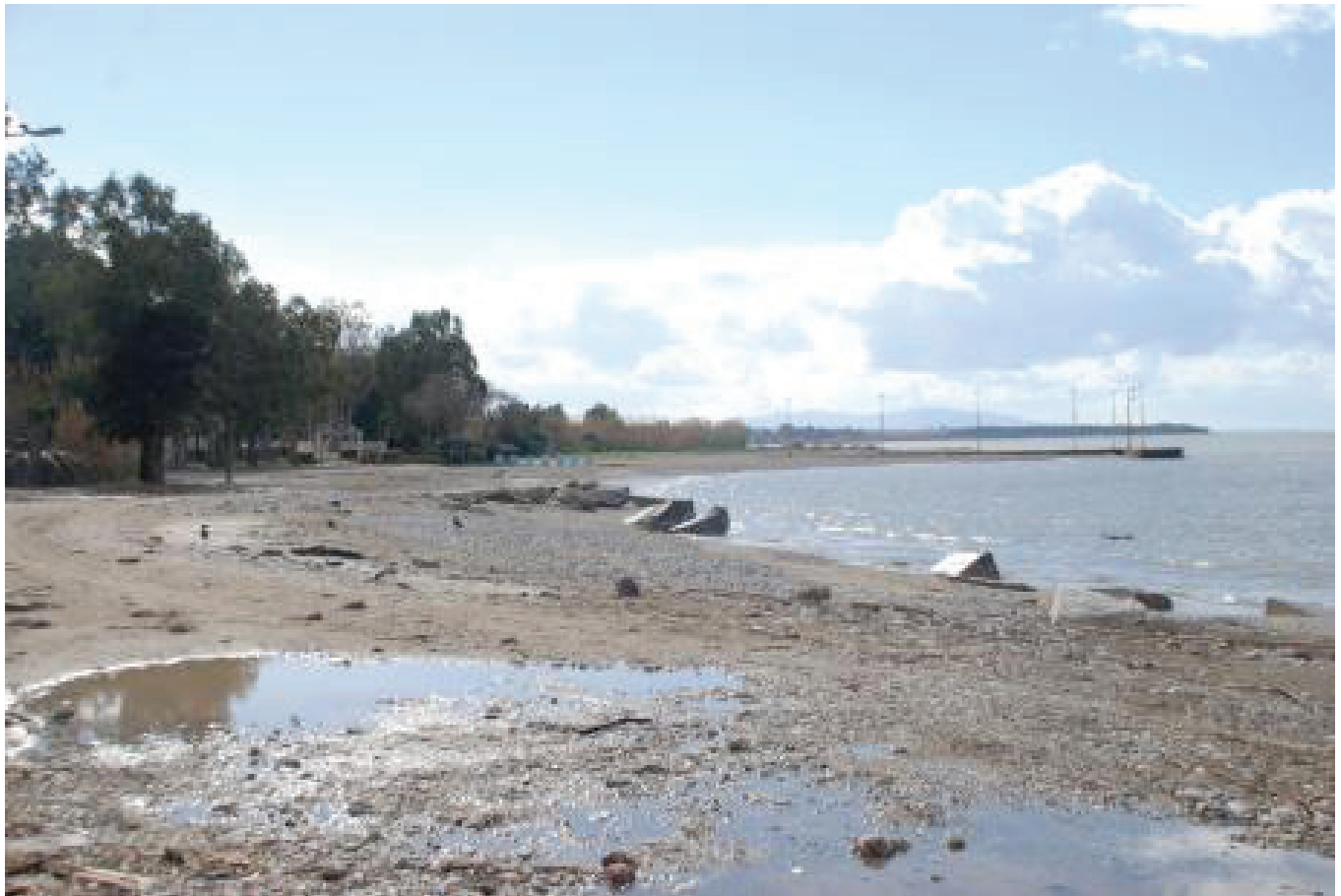
Figure 4(d) – Infrastructure and building problems in broader Rio area due to landslides, coastal erosion and poor development design.
